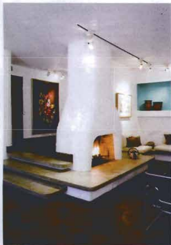
The second of three concrete steps that lead from the entry to the living room curves around itself to become the hearth of the sculptural fireplace and continues around the walls to serve as a platform for seating.
